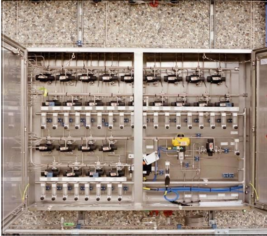
FIGURE 6. SAMPLE CONDITIONING SYSTEM FACILITATING A 26 PORT STREAM SELECTOR
